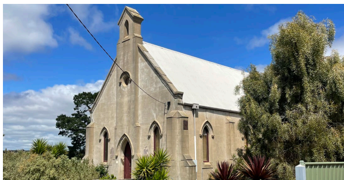
The Former St. Andrews Presbyterian Church
