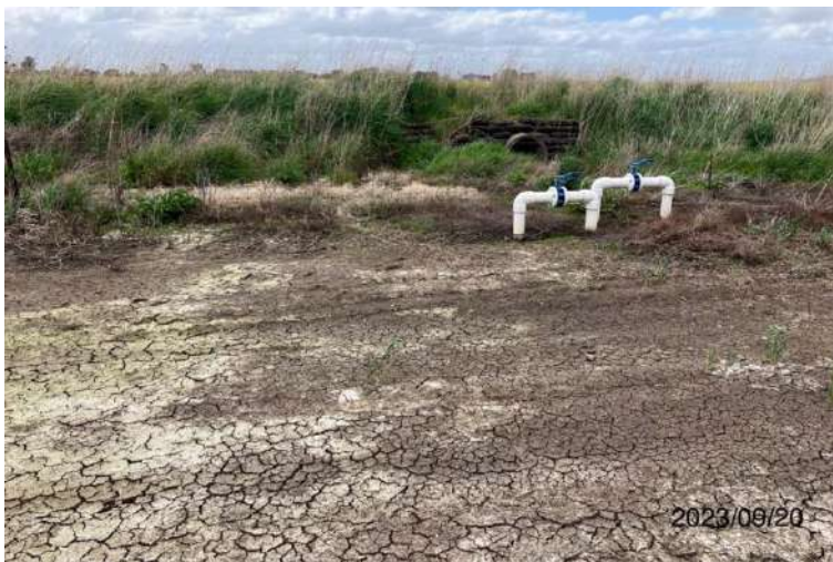
Plate 3. Degraded vegetation and crops, typical conditions, water supply pipeline.
