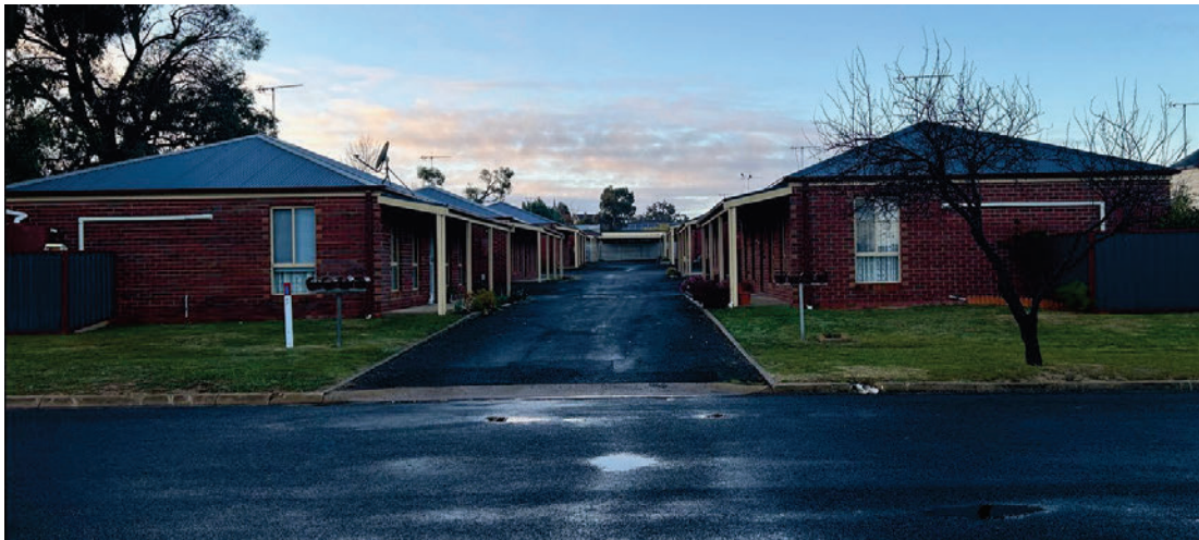
Figure 12 – 8 McKean Street (photo 12/07/24)
