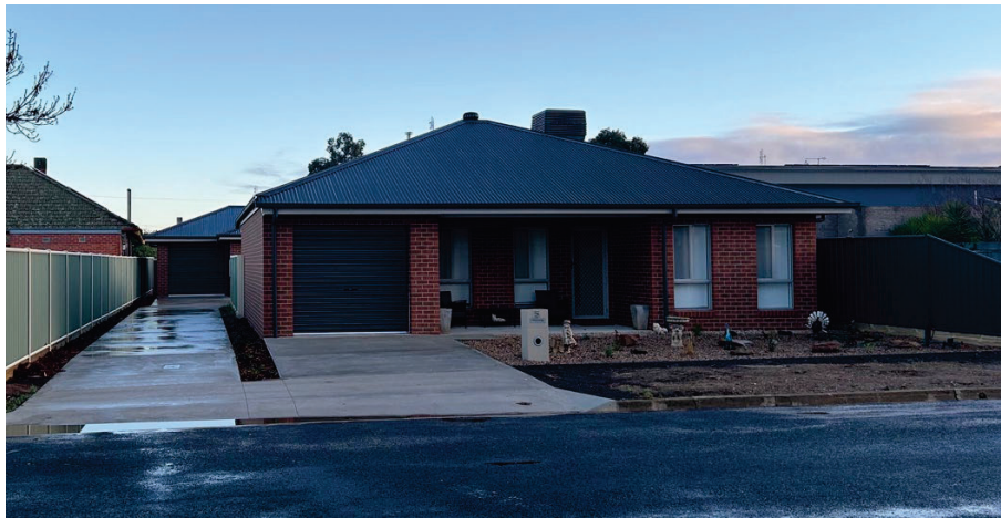
Figure 9 – 3 & 5 McKean Street (photo 12/07/24)
