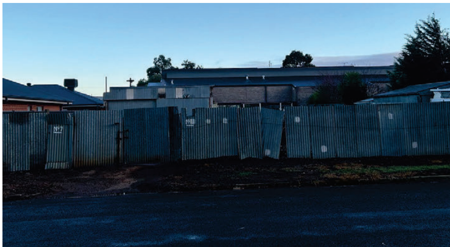
Figure 10 – 7 McKean Street (photo 12/07/24)
