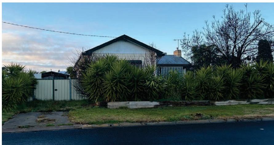
Figure 15 – 2 McKean Street (photo 12/07/24)
