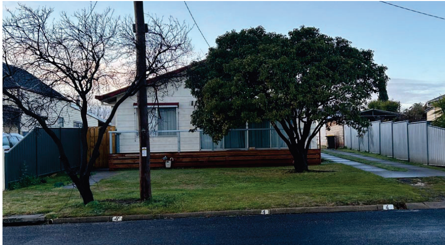
Figure 14 – 4 McKean Street (photo 12/07/24)
