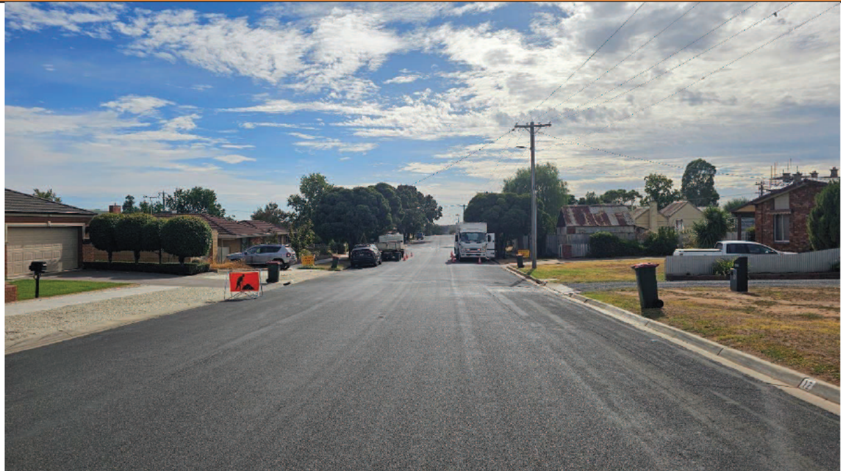
Photo 4 Looking north east along Goldsmith Street at the site entry
