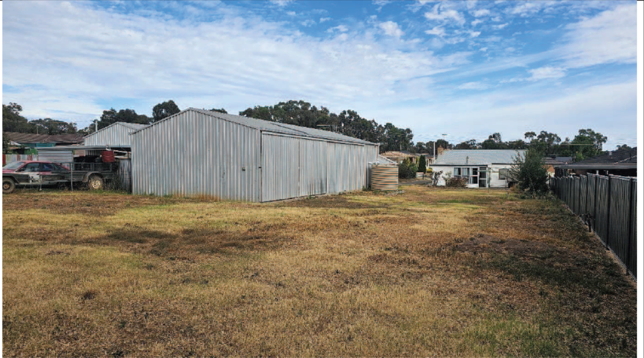
Photo 2 Looking north west from the south east boundary of the site
