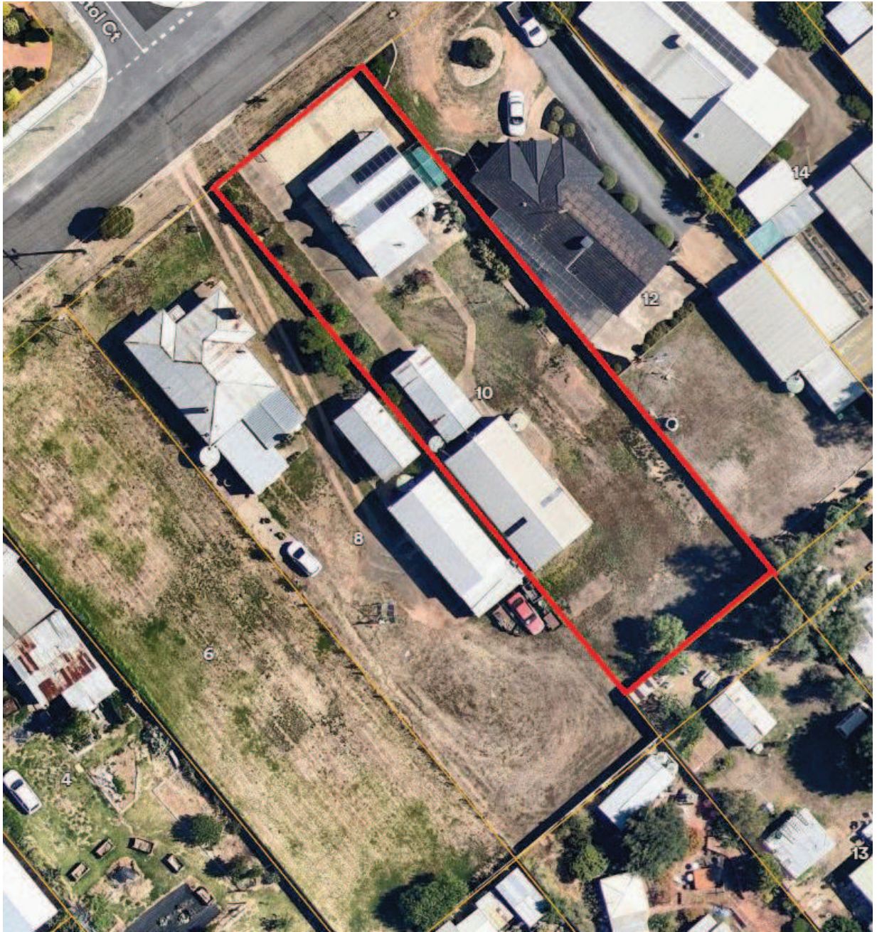
Figure 4 Existing Conditions Aerial Photo
