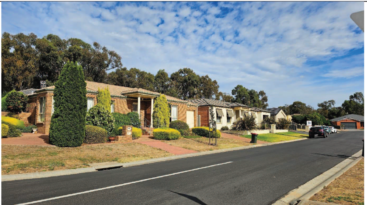
Photo 9 Looking north across managed low threat vegetation to the north east of site
