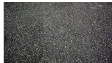
Asphalt Surfacing suitable for footpaths
