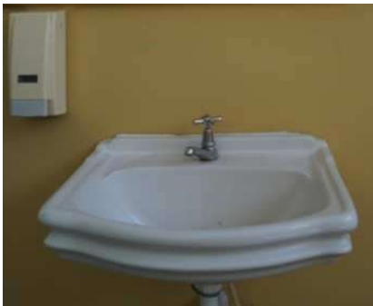
Original wash hand basin.
