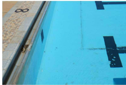
View showing the scum gutter.
