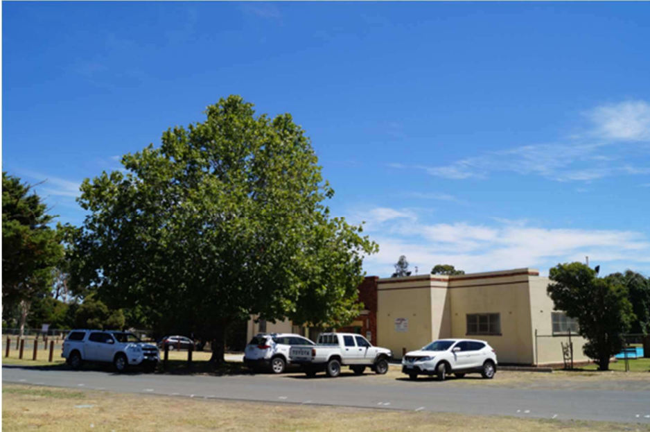
Maryborough Municipal Olympic Swimming Pool Complex 5 Lake Road, Maryborough
