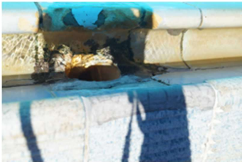
View showing the scum gutter.
