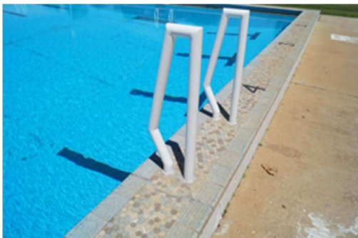
View showing the cracking along the junction of the upstand at the base and also beneath the tiles. Cracks are across the tiles and vertical.
