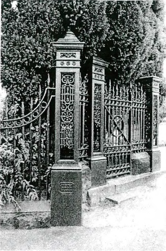
Figure 3.2a Cast iron fence and gates, north western corner of Carlton Gardens, Melbourne.
