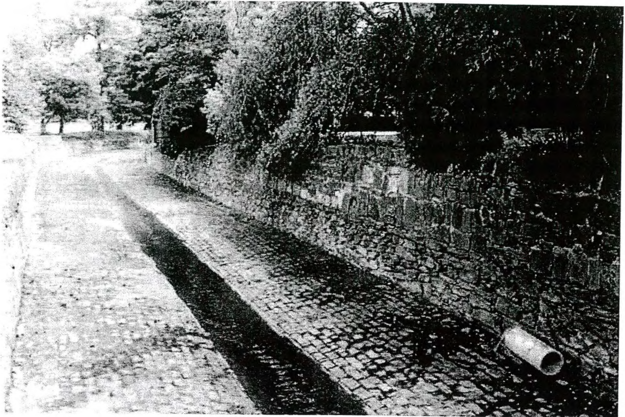
Figure 3.8 Main Drain south of main entry bridge
