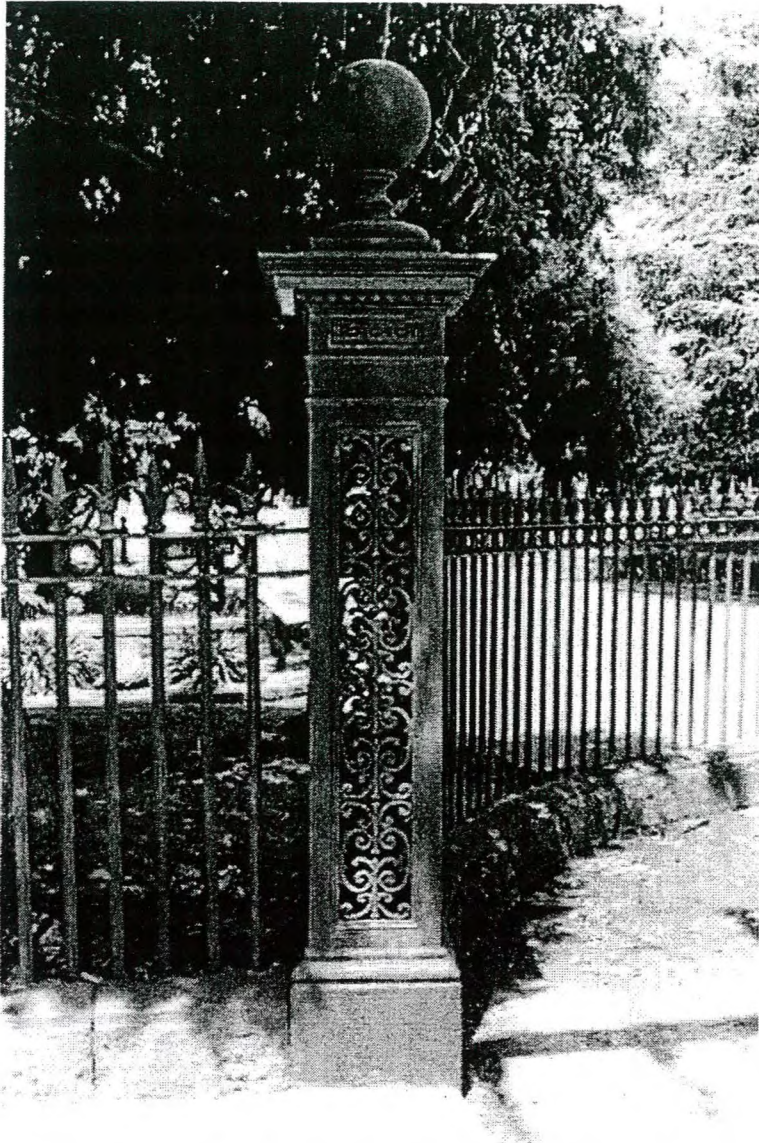
Figure 3.2 Cast iron post to the northern side of the main entrance
