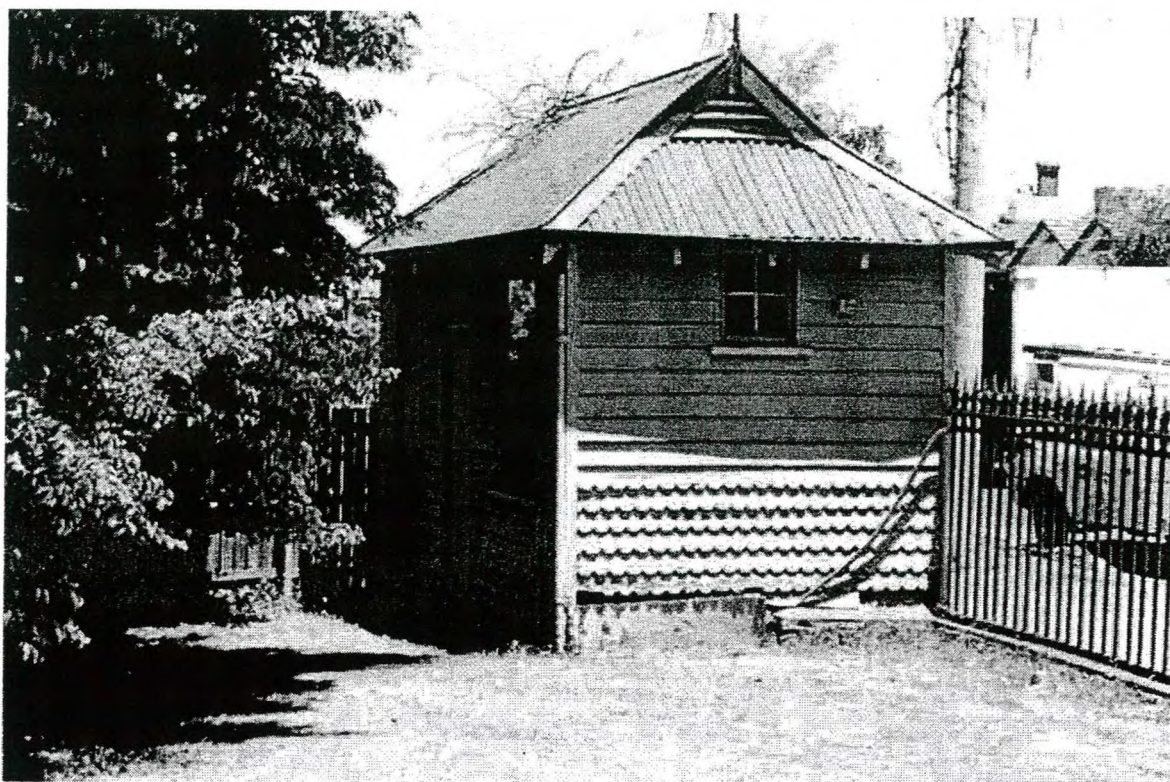
Figure 3.4 View of ticket office from north east.
