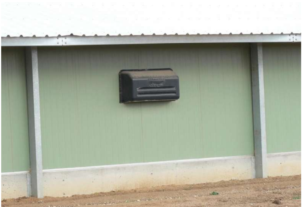
Photo 6: Typical mini vent (external wall)
