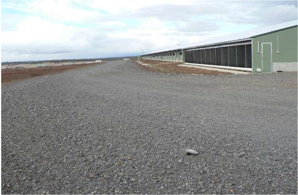
Photo 3: Side wall of broiler shed
