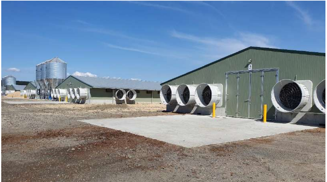
Photo 1: Typical broiler sheds (fan end)
