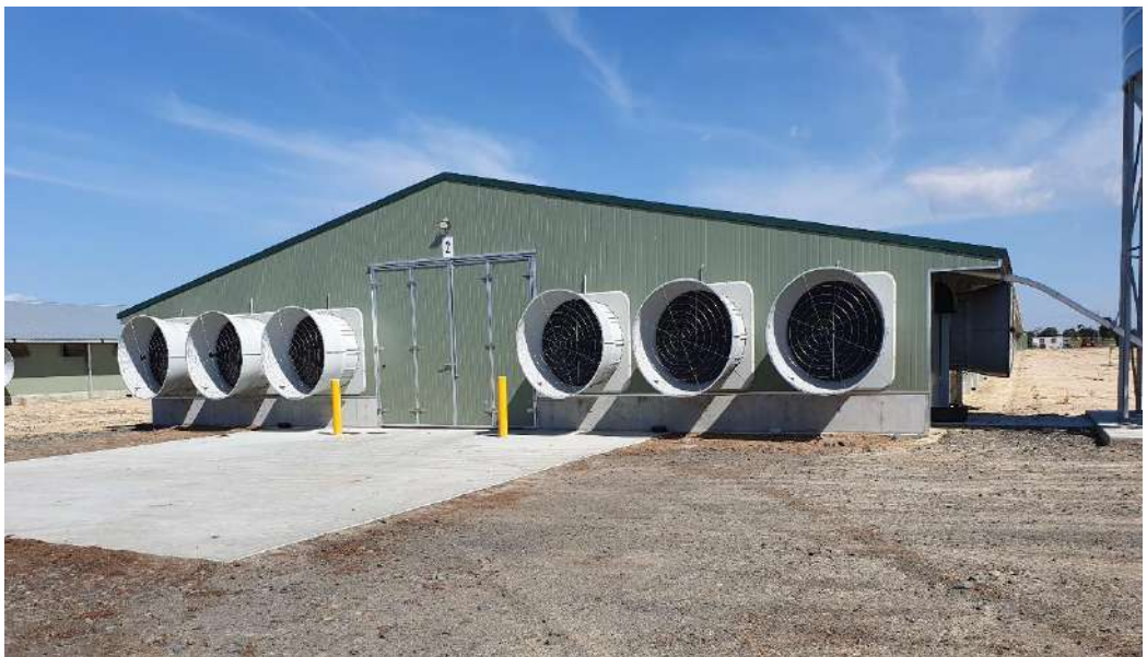
Photo 4: Typical end of shed showing fans
