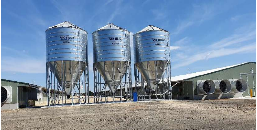
Photo 7: Typical feed silos
