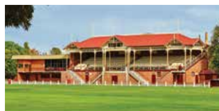
Princes Park Grandstand
