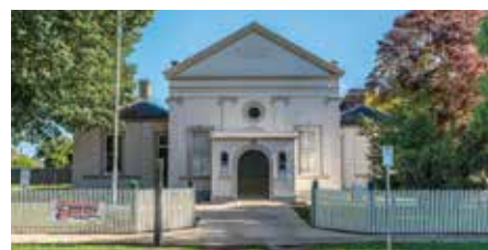
Town Hall Restoration Package (Maryborough Town Hall, Carisbrook Town Hall)
