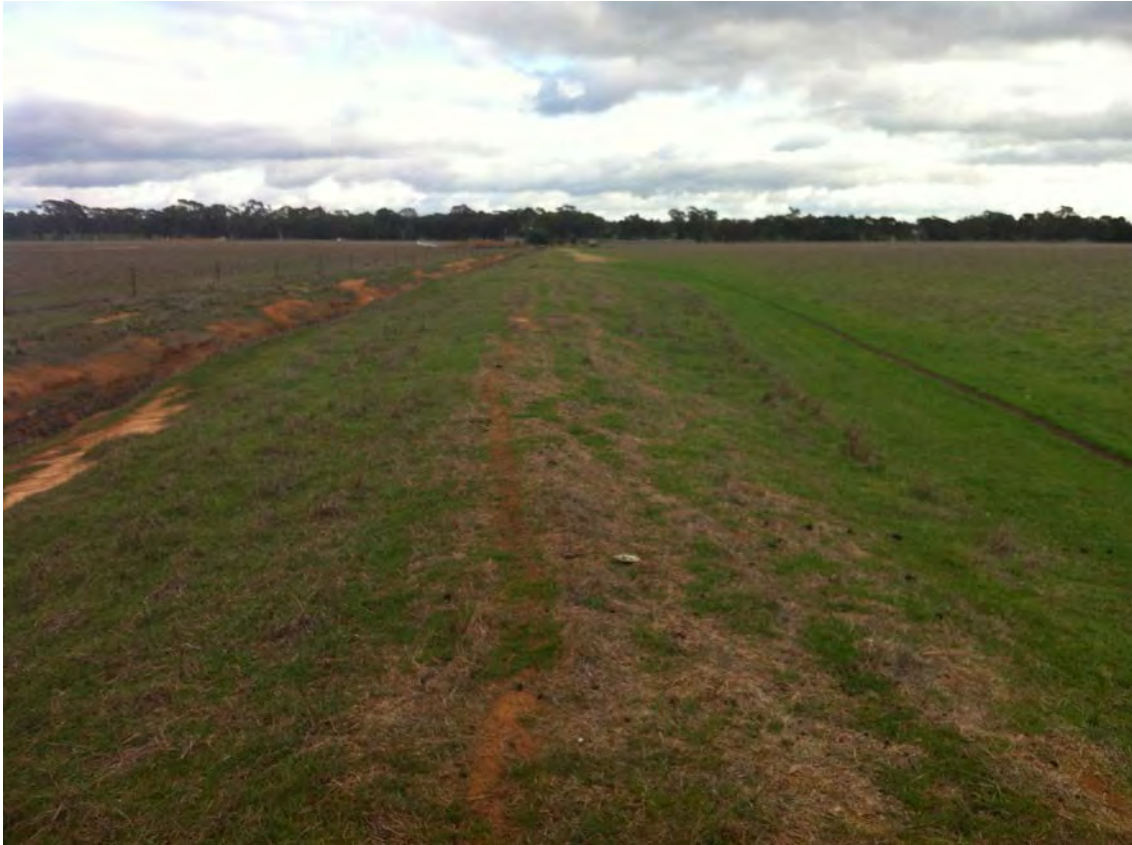
Figure 3. Existing drain, proposed for levee construction.
