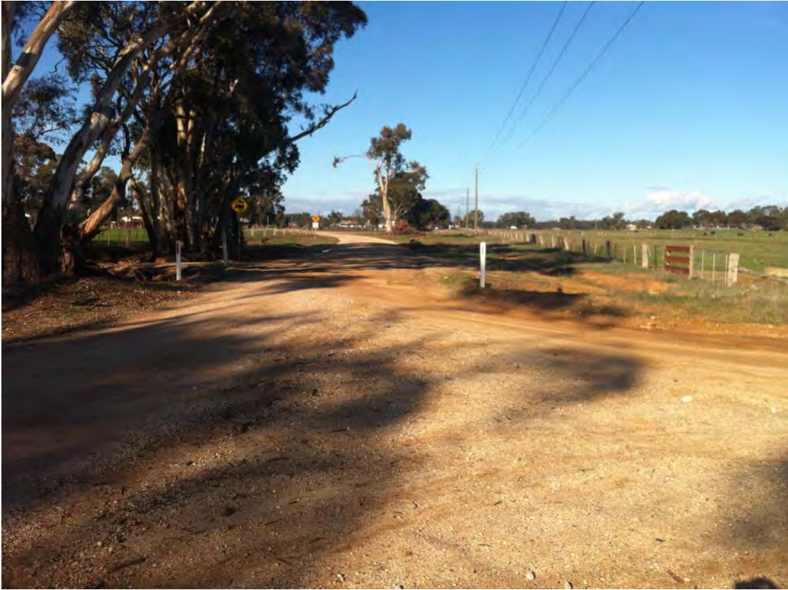
Figure 1. Pleasant Street, Carisbrook, proposed for levee construction.
