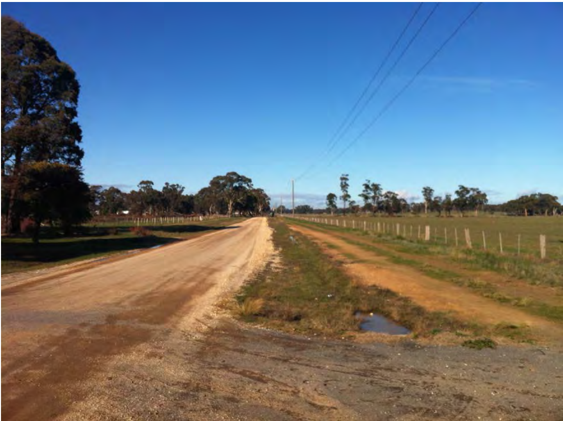
Figure 2. Pleasant Street, Carisbrook, proposed for levee construction.
