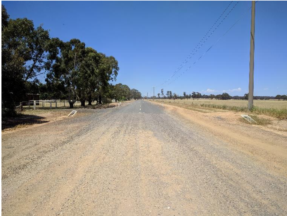
Figure 4.7 : Western levee along Pleasant Street at (approx.) chainage 2700m looking south
