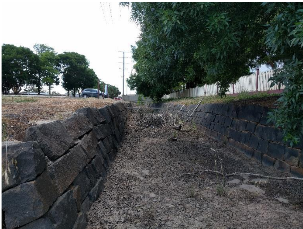
Figure 4.2 : Bluestone drain near corner of Camp Street and Landrigan Road
