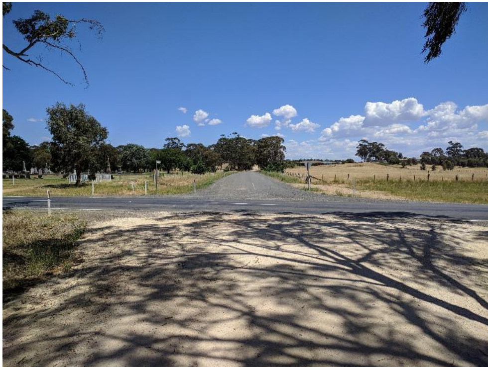
Figure 4.4 : Williams Road Levee at the junction of Williams Road and Landigan Road looking west
