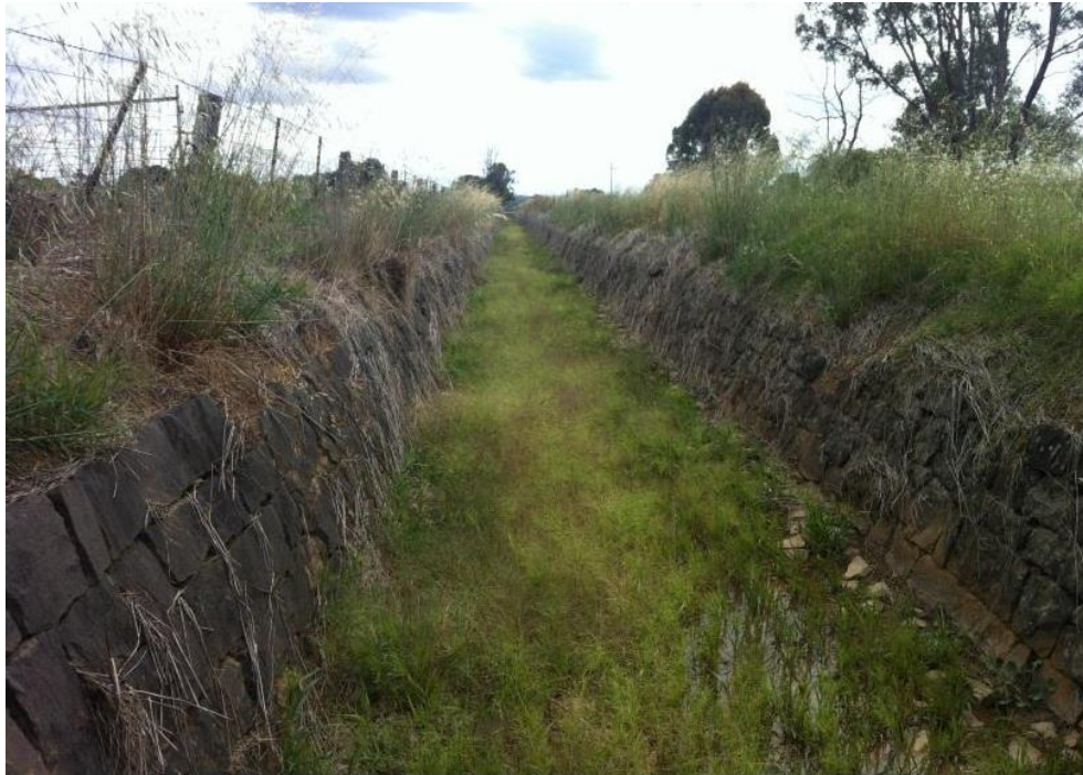
Figure 4.3 : Bluestone drain near Hood Street
