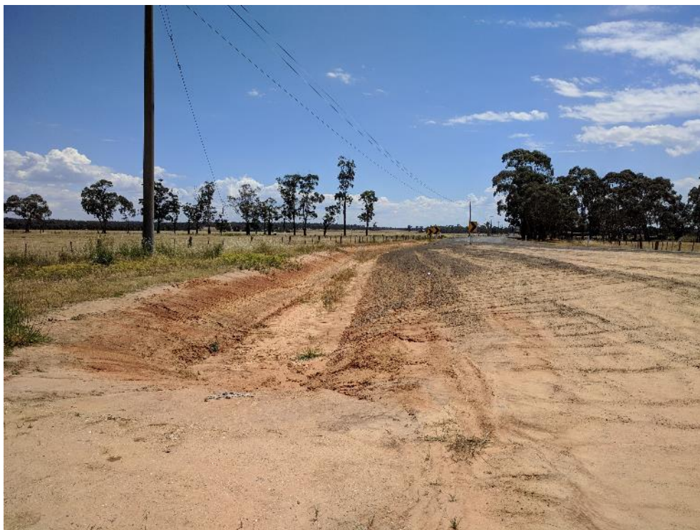
Figure 4.8 : Drain along western side of the levee
