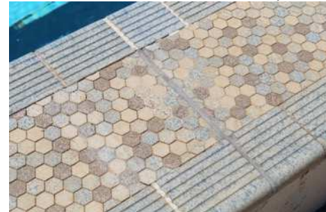
Continuous crack repairs where the tiles have substantially moved apart.
