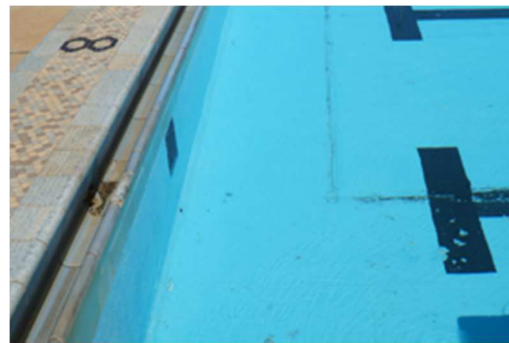
View showing the scum gutter.
