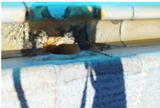
View showing the scum gutter.
