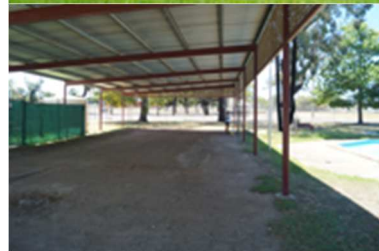
View of the interior of the shelter.
