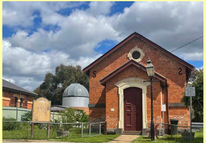
Free Library Building
