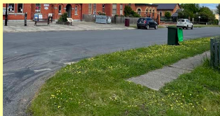
Disconnected paths (Camp Street)
