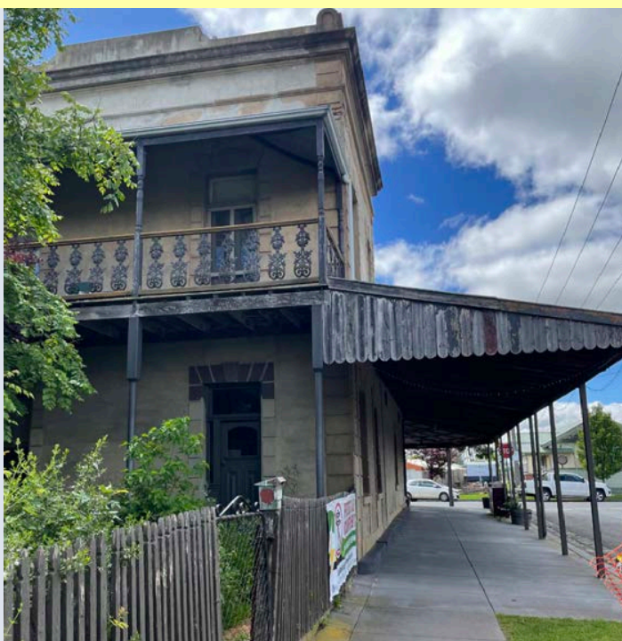
Two storey form on the corner of Camp Street & Scandinavian Crescent
