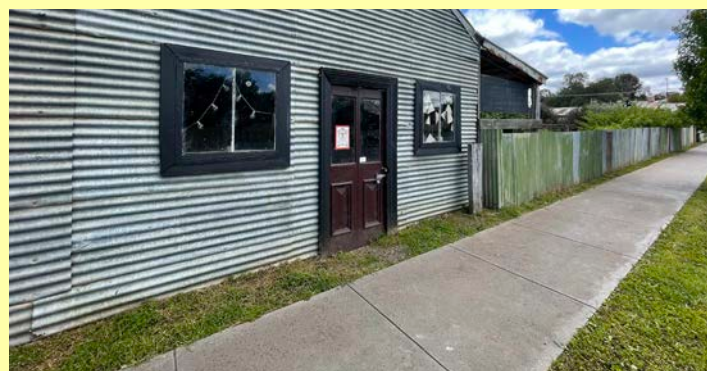
Scandinavia Crescent footpath (outside core area)
