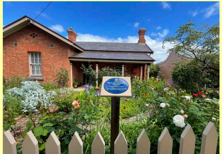
Former Talbot Police Residence & Lock-Up
