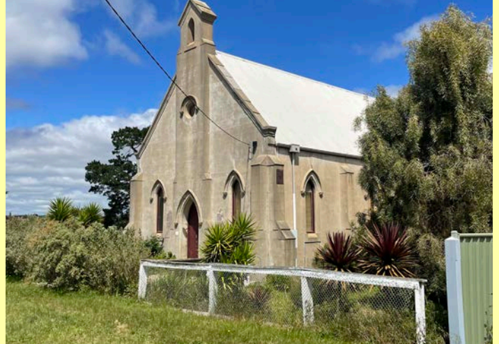
The Former St. Andrews Presbyterian Church
