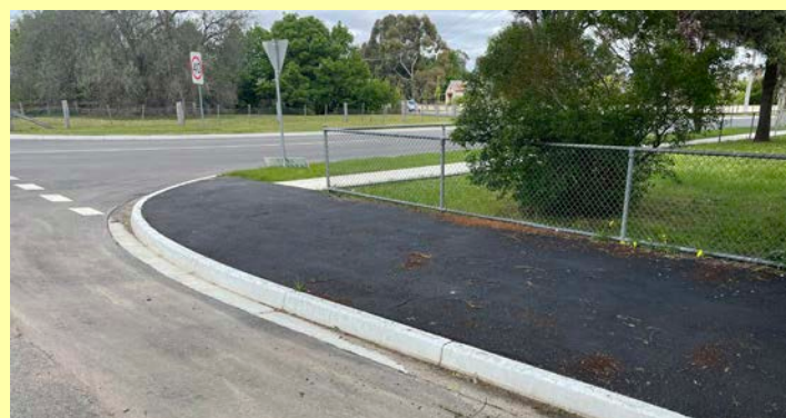
New footpath outside Talbot Primary School
