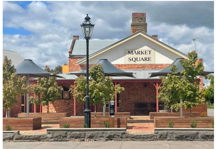
The outdoor space at Market Square
