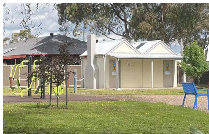
Pioneer Park with public toilet and new gym equipment
