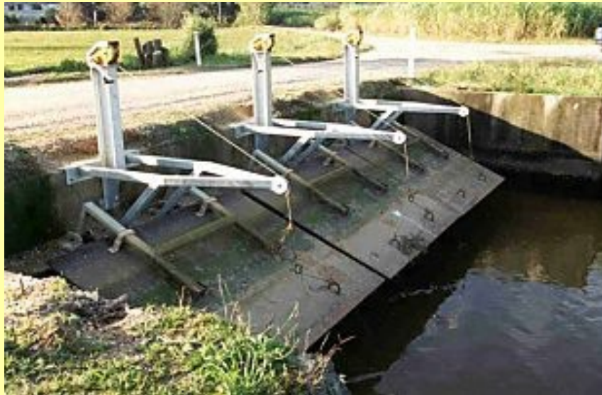
Figure 4-35 Lifting Arm on Flap Valves
