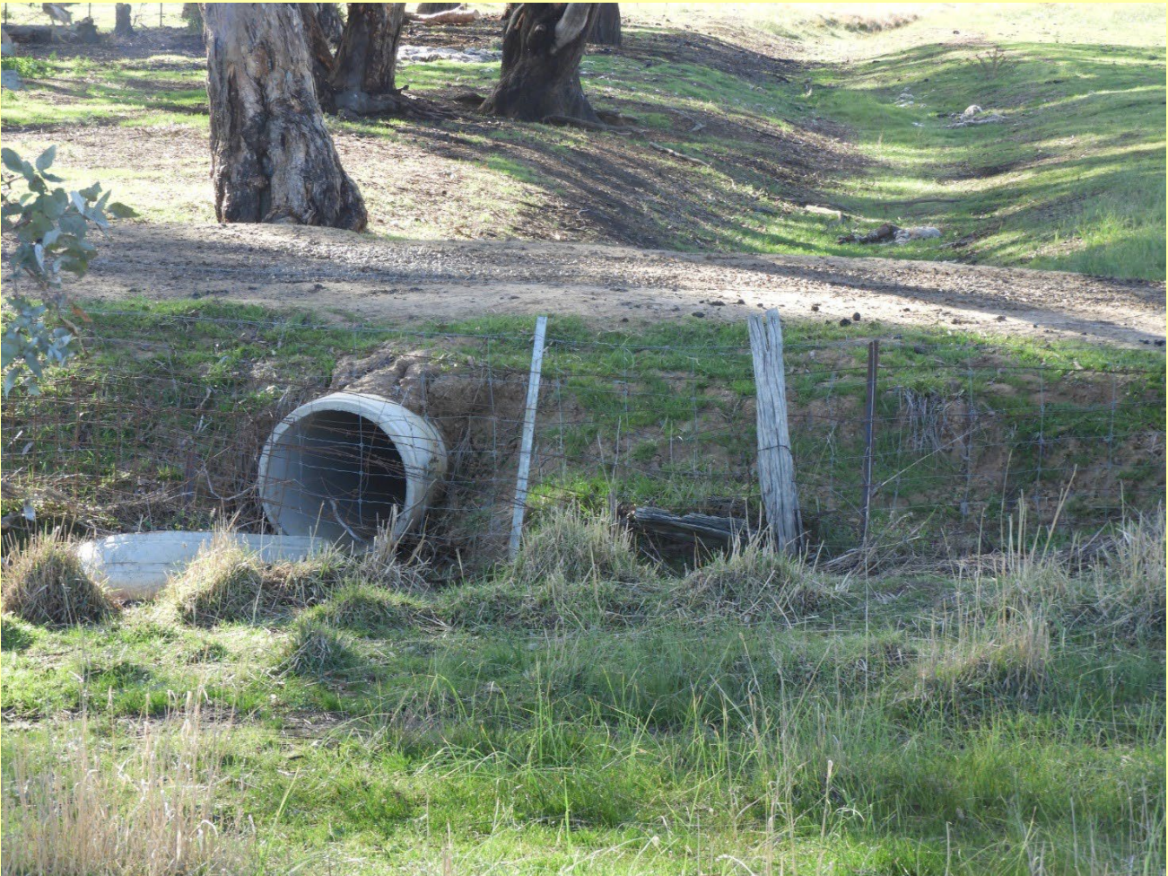
Figure 4-23 Block bank and pipe north of railway line west of Pleasant and High Street
