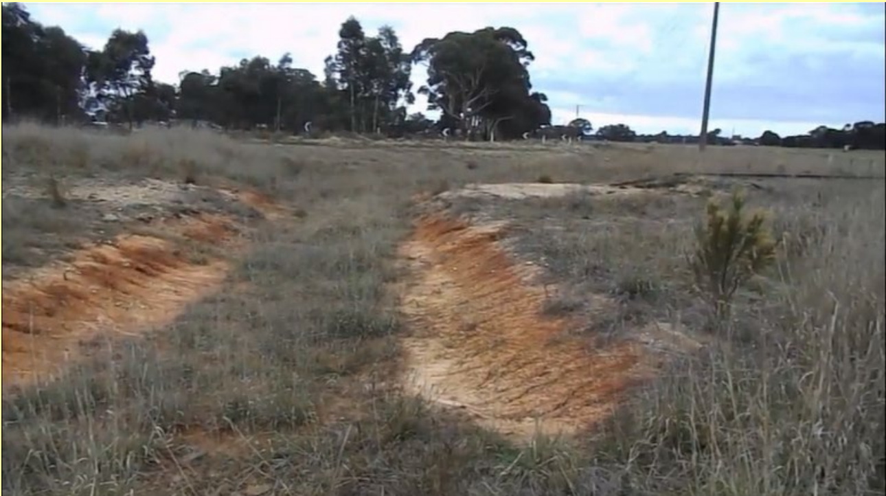
Figure 4-21 Channel through cutting in railway line near Pleasant and High Street
