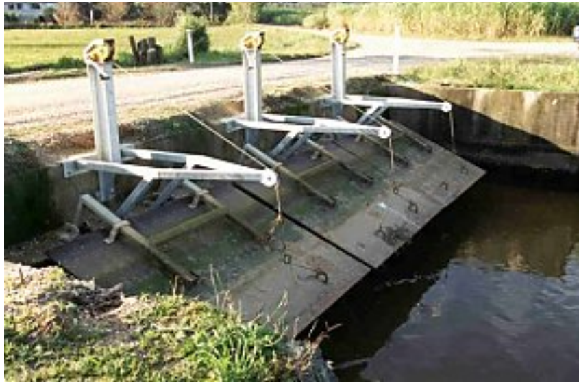
Figure 4-35 Lifting Arm on Flap Valves
