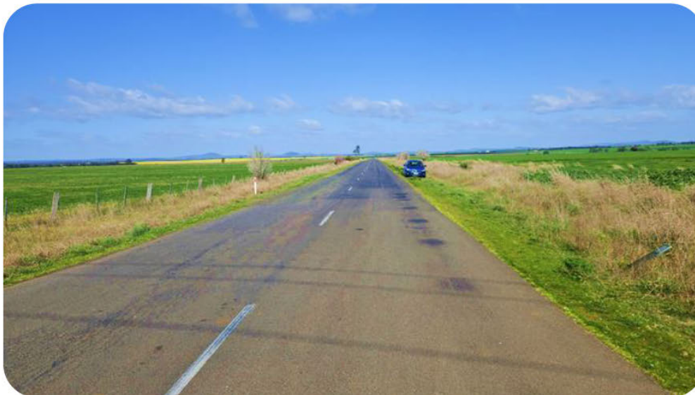
Figure 6 Typical View of Locks Lane
