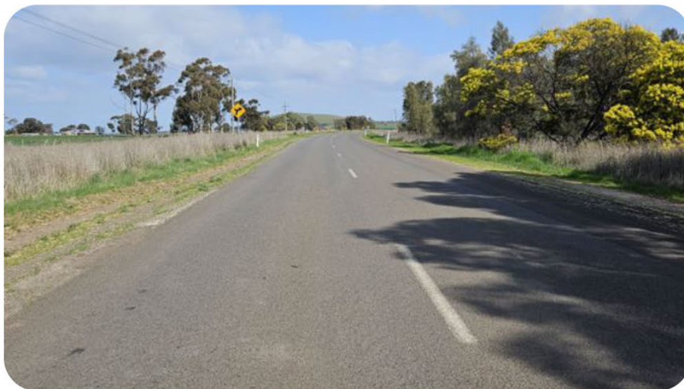
Figure 8 Typical View of Baringhup Road
