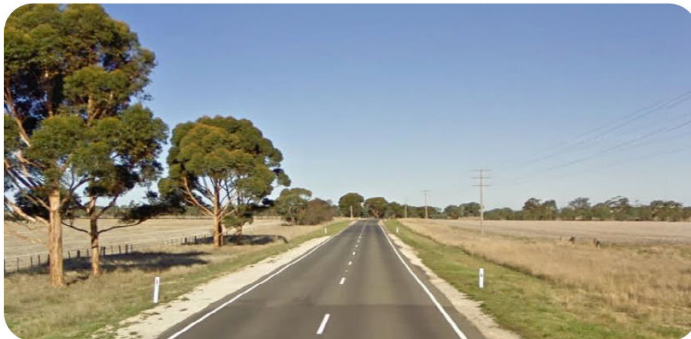
Figure 3 Typical View of Pyrenees Highway
