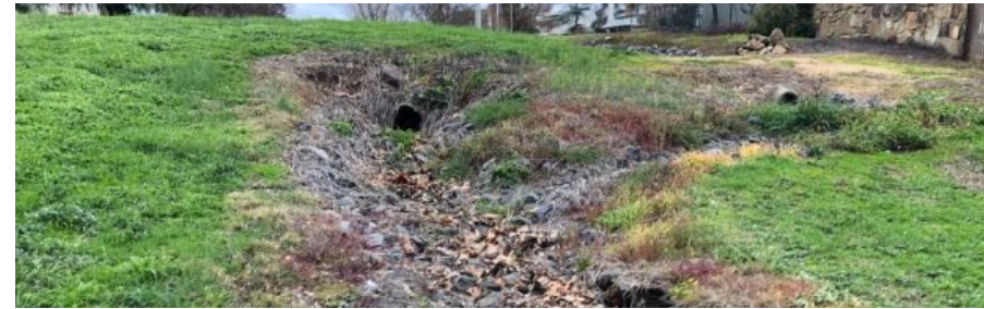
Figure 2-5: Stormwater outfall off McNeil Street
