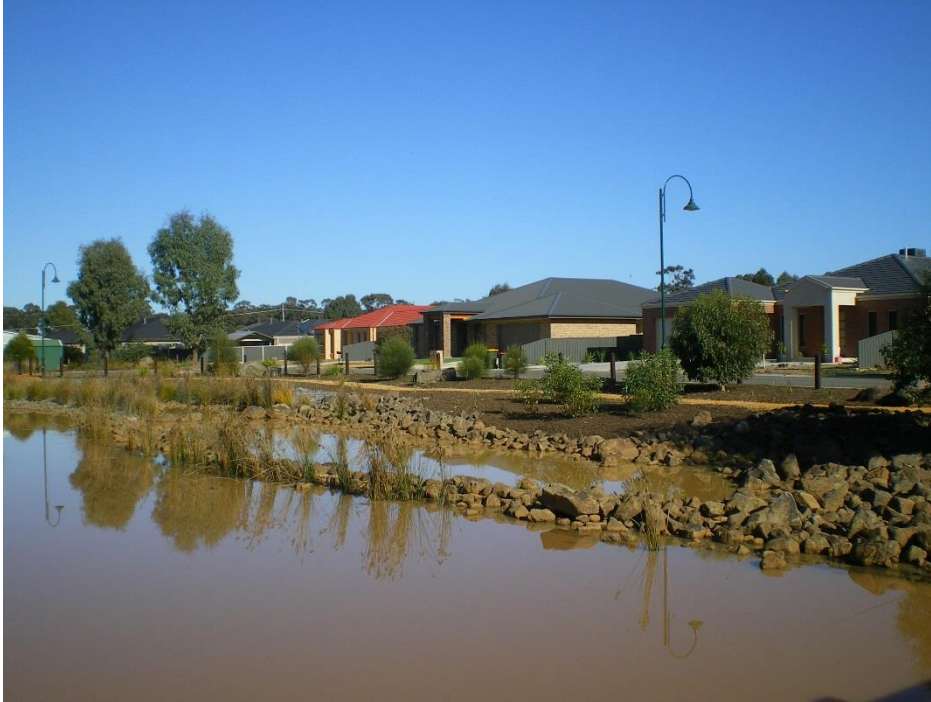
Part of the Whirakee Rise development within Maryborough
