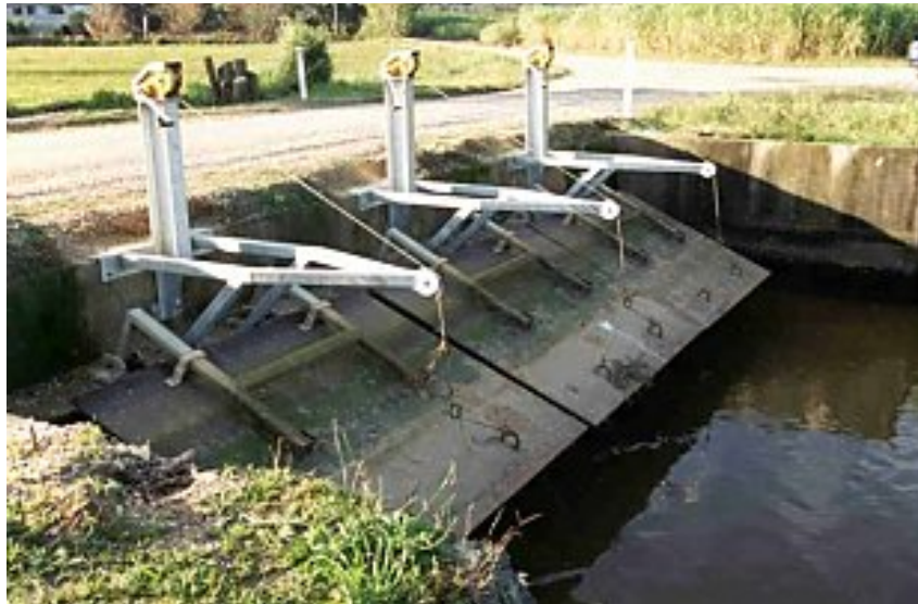
Figure 4-35 Lifting Arm on Flap Valves
