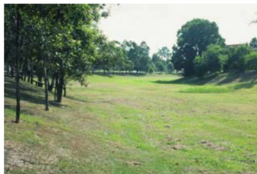
Figure 4-25 Photo of channel with manning's roughness GREATER than 0.022
