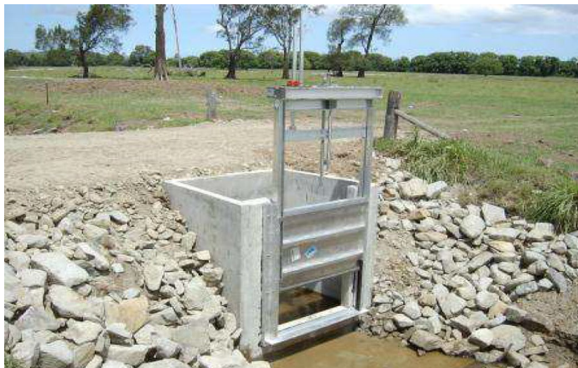
Figure 4-36 Example of Sluice Gate Valve
